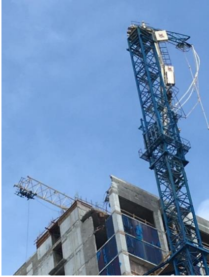
The construction crane at Vice in downtown Miami snapped during Hurricane Irma.
